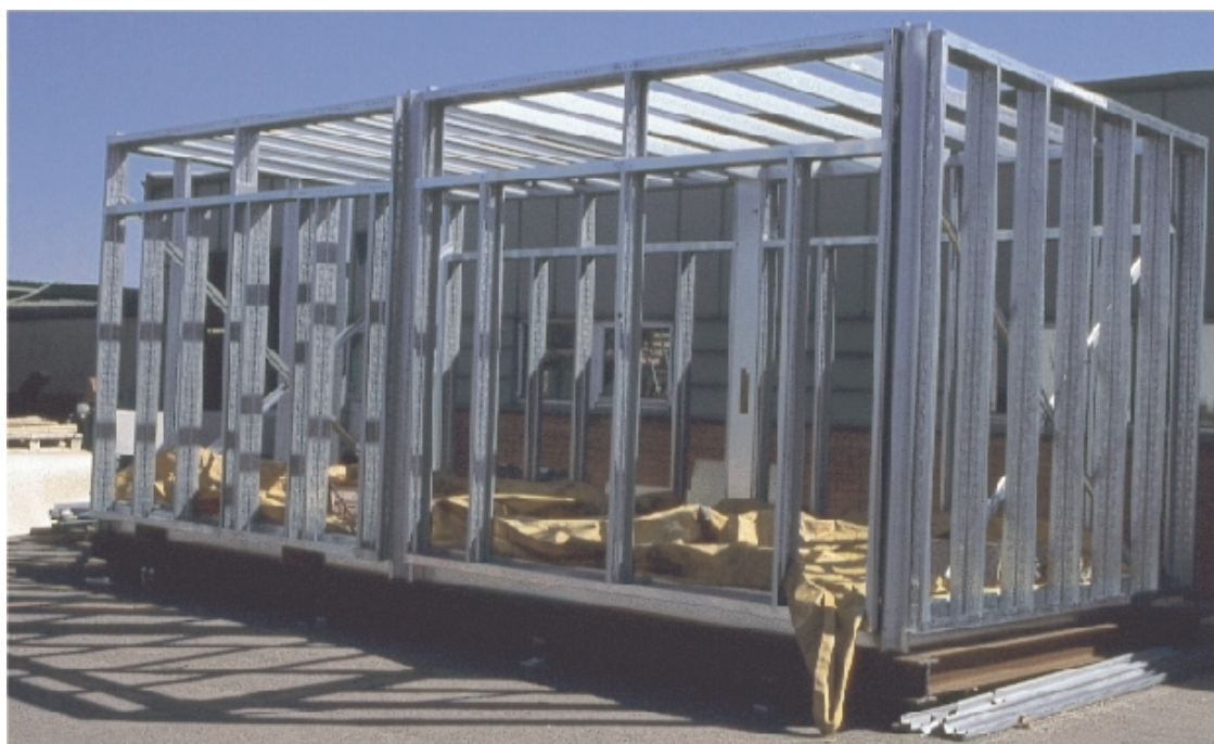
Figure 3: A light-gauge steel frame for modular housing units.
